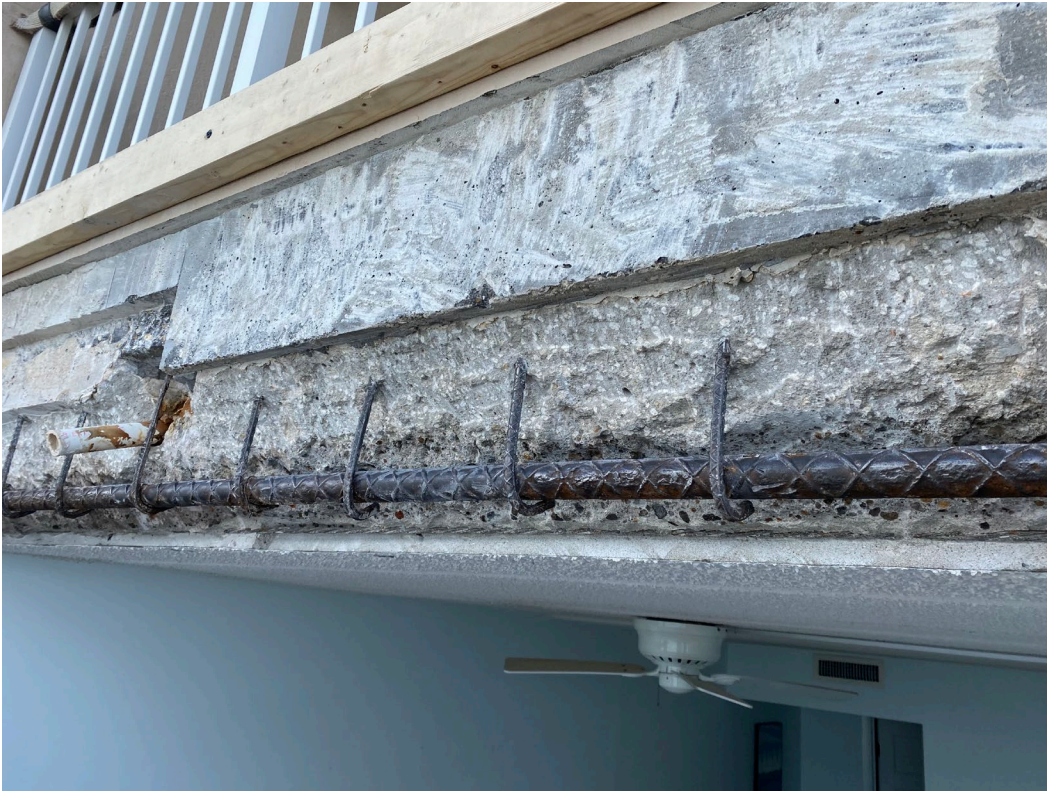
Picture 1: Unit 692 window header repair
