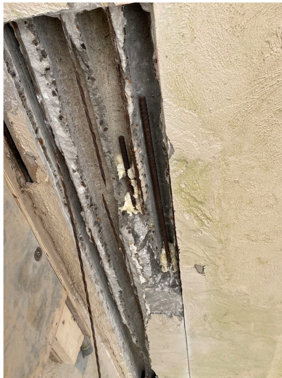
Picture 2: In-progress walkway repair
