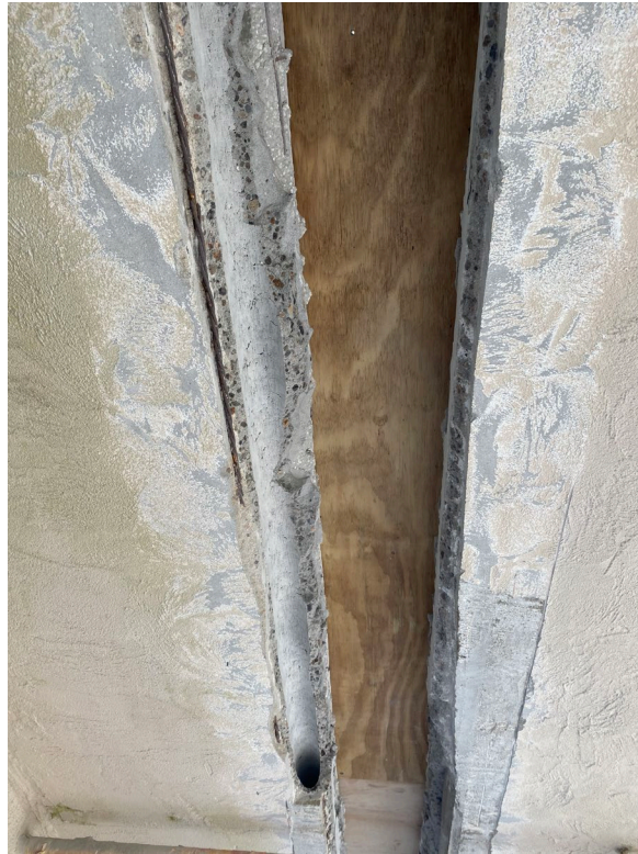
Picture 3: In-progress walkway repair
